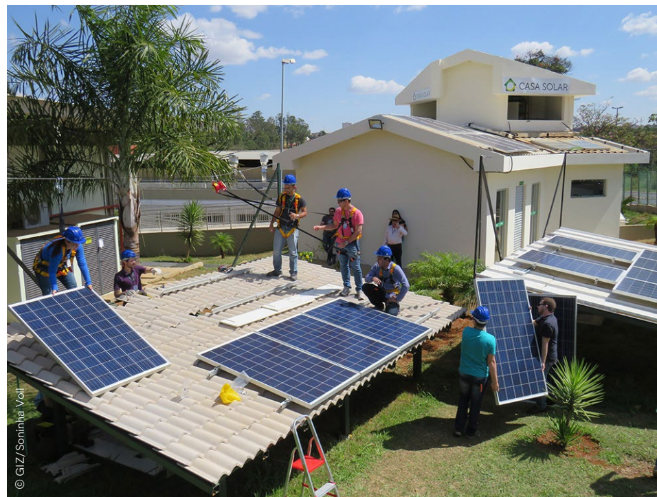
Installing solar panels to generate electricity necessary for the production of green hydrogen
