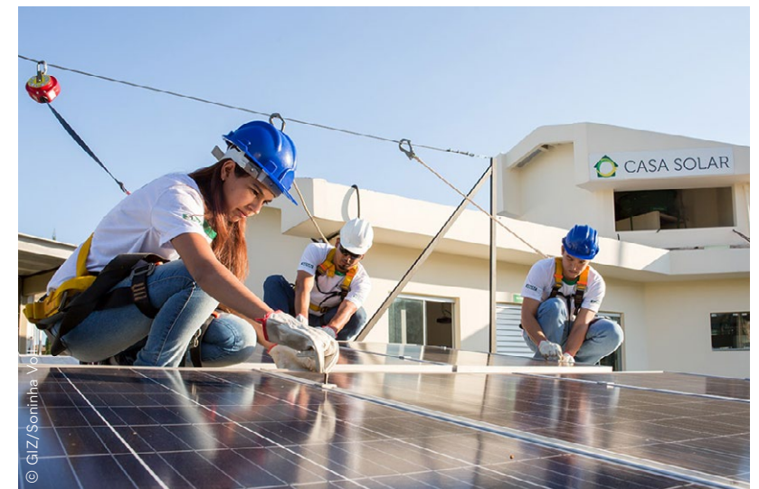
Installing solar panels to generate electricity necessary for the production of green hydrogen
