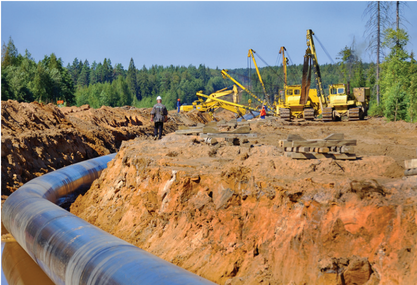
Image 7. Construction of a gas pipeline
