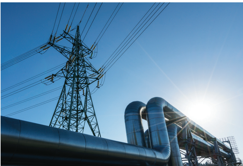
Image 11. The gas and electricity industries often intersect, leading to an often unclear distinction between trades
