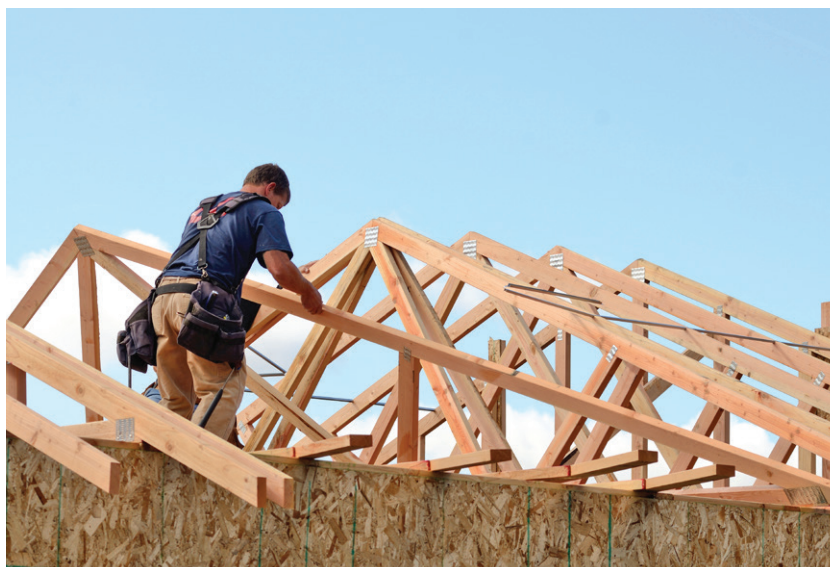
Image 12. Construction workers will be required to support the development of hydrogen buildings
